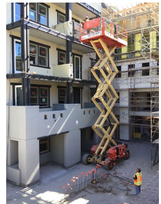
Building C from Courtyard View
