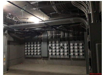
Garage Meter Room B Installations Completed
