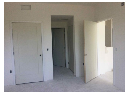
Door and Door Trim Installation in Building C unit
