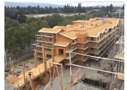
View of Building B and Bridge
