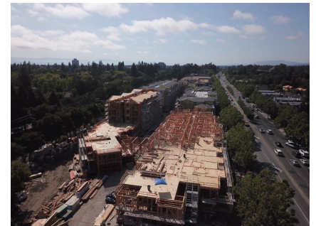
Aerial View of Construction Site
