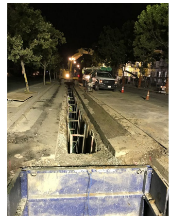
Sanitary Sewer Connection Work on El Camino Real
