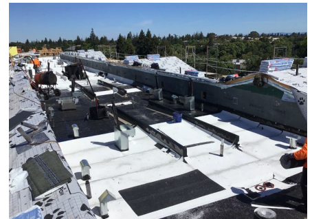
Installing Roof Membrane at Bldg B
