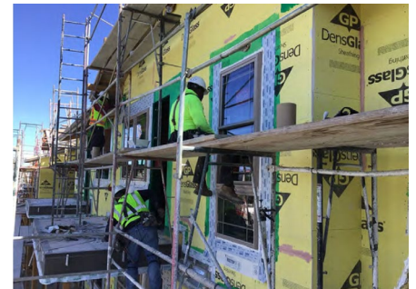
Window Installations at Building B
