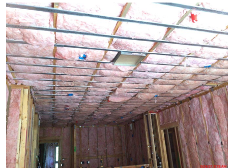
Completing Residential Insulation
