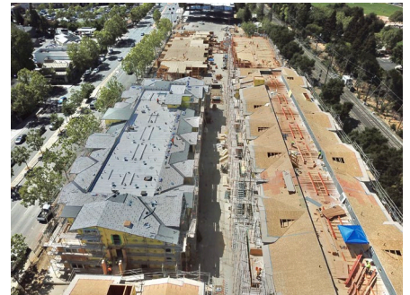
Aerial View of Construction Site
