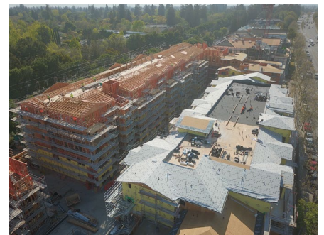
Aerial View of Construction Site
