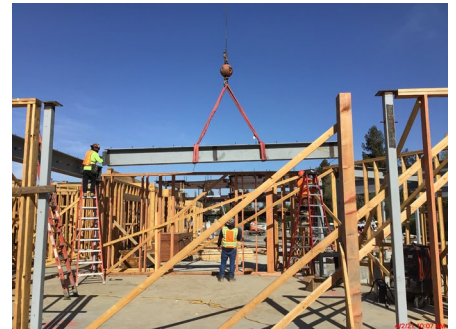
Hoisting of Structural Steel at Building A
