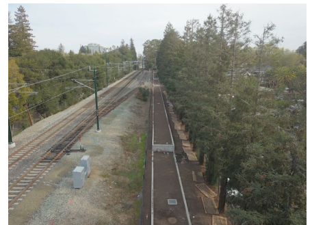
Bioswale Soil Placement Complete
