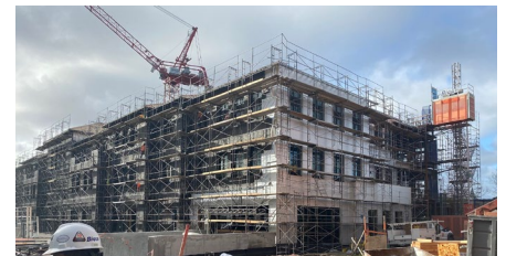
Stucco Preparation at Office Building 2
