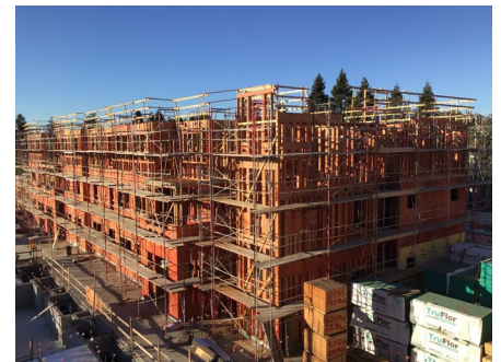
3 rd level framing of Building A
