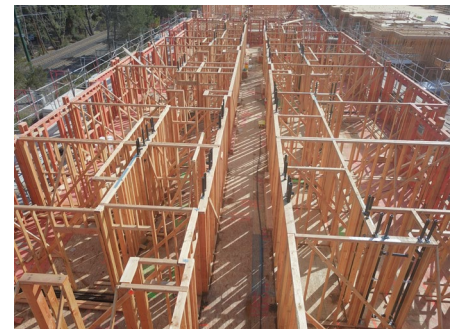
2nd Level Building Framing In Progress
