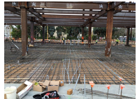
Installation of Reinforcing Steel
