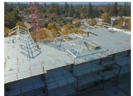
Steel Structure Erection
