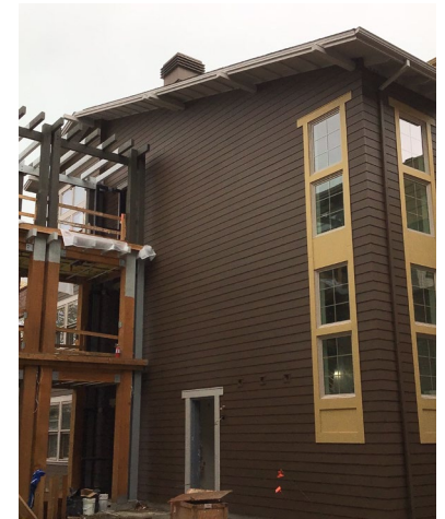
Residential Bridge Construction & Exterior Paint Progress
