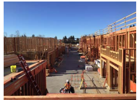
Upper level framing in progress
