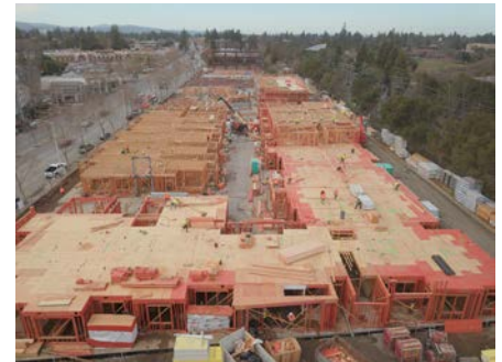
Aerial view of construction site
