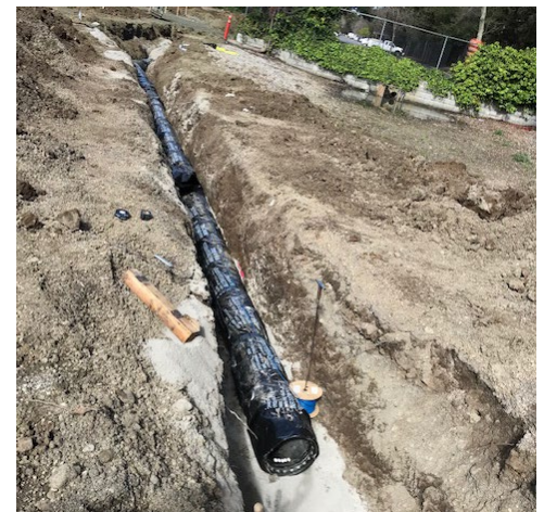
Cal Water Pipe Trench
