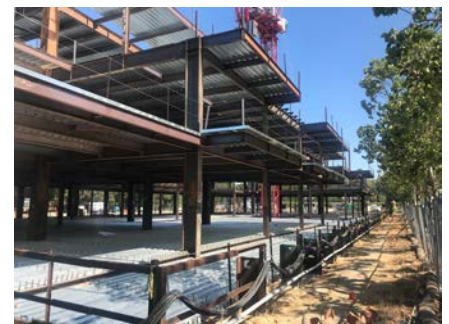
Office Building 2 Steel Structure
