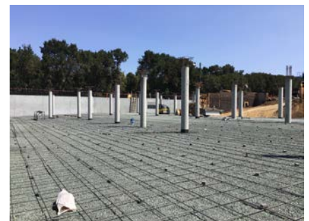
Foundations Preparation for Concrete Pours
