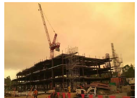
Office Building 2 Steel Erection
