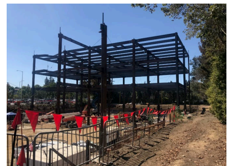
Office Building 1 Steel Structure
