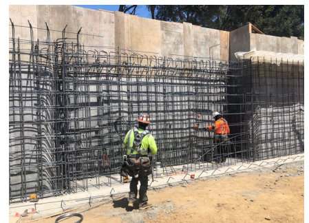
Building B Wall Rebar
