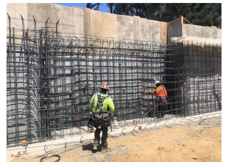
Building B Wall Rebar
