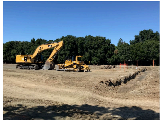
Site Preparations Continue
