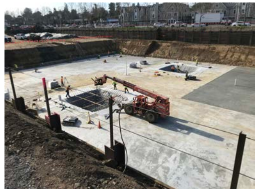
Site Preparations Continue
