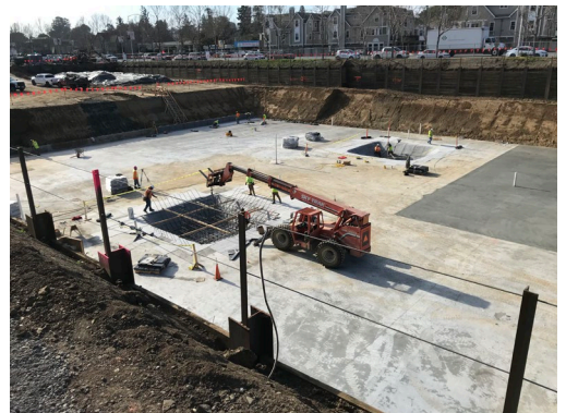
Site Preparations Continue
