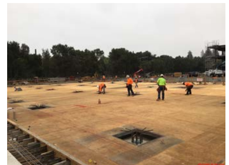
Level 1 Parking Structure
