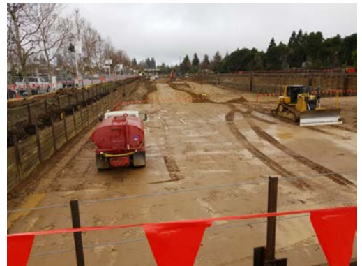
Site Preparations Continue
