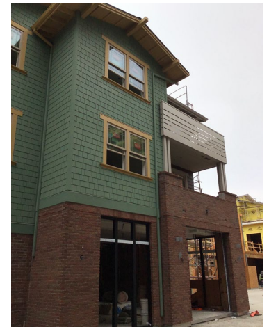
Section of Building C Exterior Complete
