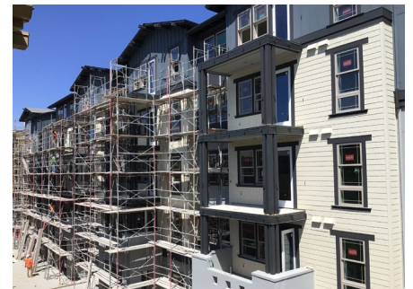
Exterior Paint Work on Residential Building B
