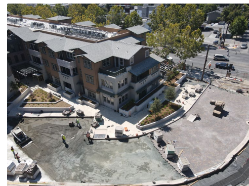
Pavers Installation by Building A
