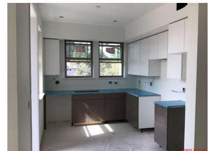
Finishing touches on Building C Interiors
