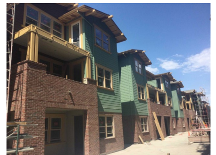
View of Building C from Courtyard
