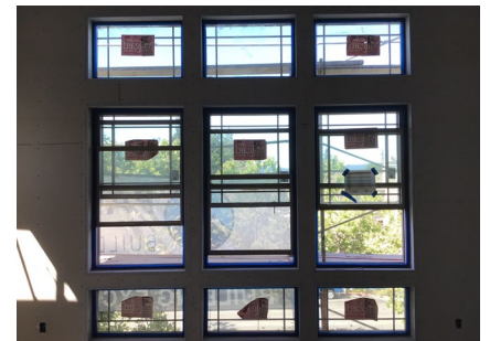
Residential Window Installation
