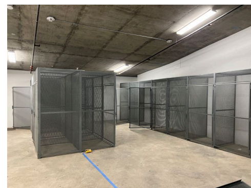
Garage Level G2 Storage Lockers
