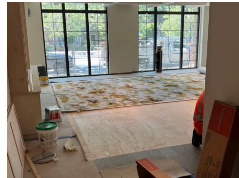
Carpet Rollout in Building C Meeting Room
