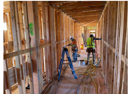
Shim and Shave of Building B Corridor
