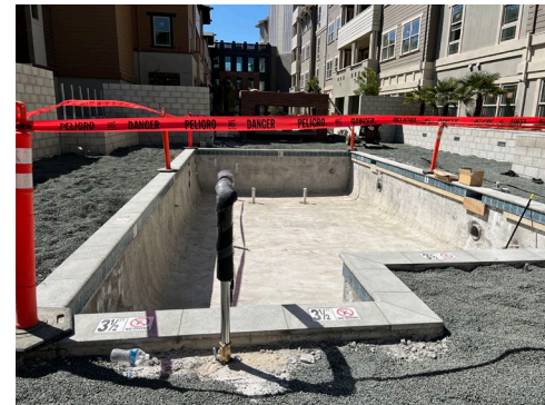
Pool Construction in Progress
