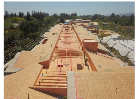
Aerial Photo of Building B Roof Sheathing and Crickets
