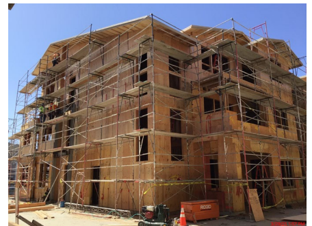
Building C Framing Nearing Completion
