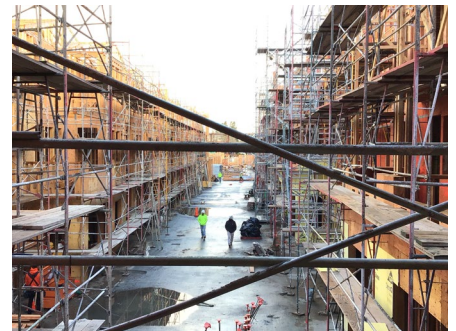
Temporary Scaffolding for Construction Access
