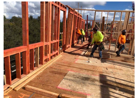
Completing Upper Level Residential Wall Framing
