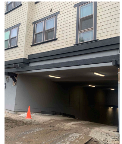
Paving of Garage Entrance
