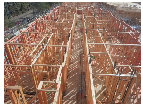
2nd Level Building Framing In Progress
