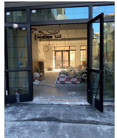
Installing Egress Doors at Lobby/Lounge in Building B
